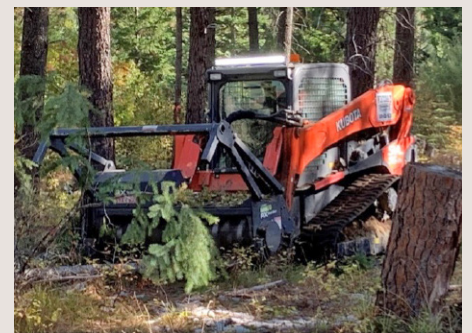
Masticators grind up small trees and underbrush.
